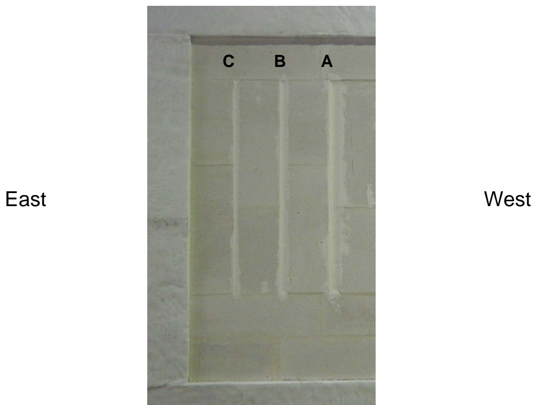
Figure A6.2: Exposed face of specimen before commencement of the fire-resistance test
