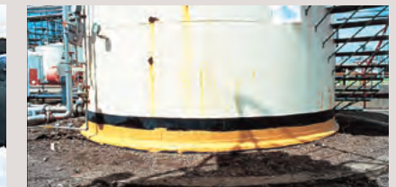
Anti-corrosion around the base of tanks.
