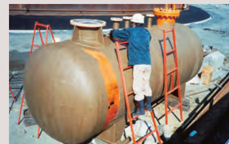
Anti-corrosion for outside of underground tanks.
