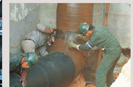
Anti-corrosion of buried steel coolant pipes.
