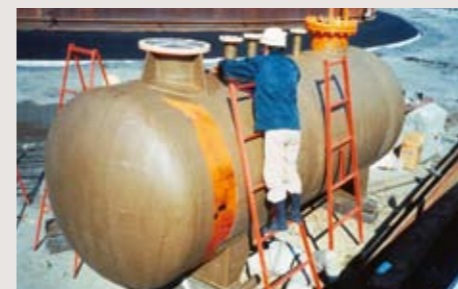
Anti-corrosion for outside of underground tanks.
