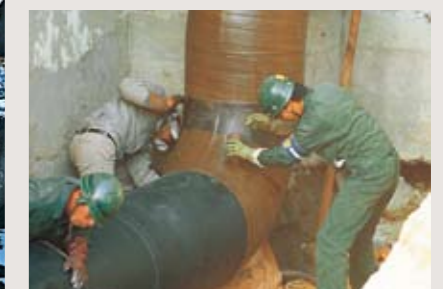
Anti-corrosion of buried steel coolant pipes.
