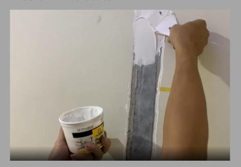
Putty Filler is an easy-to-use multi-purpose filler specially formulated to fill cracks and gaps in a single application. It has virtually no shrinkage and is smooth and durable. It is paintable with oil and water based paints.
