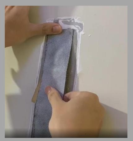
No. 6931 is a self-adhered, waterproofing airtight tape designed for sealing building joint areas. This product has a butyl rubber adhesive that offer superior adhesion durability
