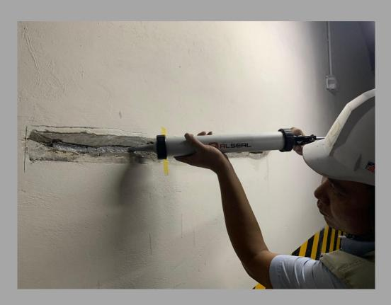
This MS sealant can accommodate +-50% movement and secure excellent bonding, paintable, permit application of Nitto Tape NO.6931 onto it.
