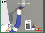
Apply RHINOZ Primer Bonding along jointing for about 3 cm width on both sides of jointing. Leave it to dry 10-15 minutes, or until the primer bonding become clear color.
