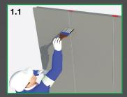
Clean the surface to be free from dust, grease and other contaminants. In case the gap is deep and wide, can install backing rod first.
