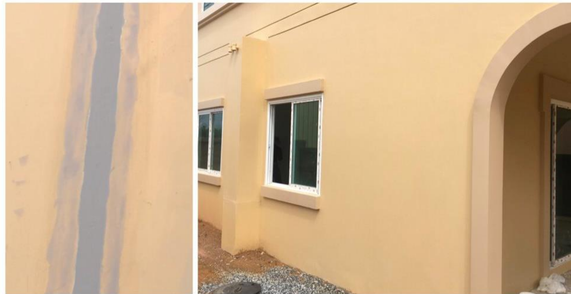
Apply RHINOZ Hybrid Jointing Compound, special formula of modified polyurethane and epoxy.
