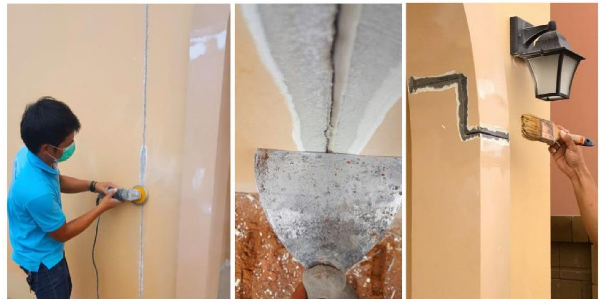
Cracks along jointing of precast panel from structure movement.
