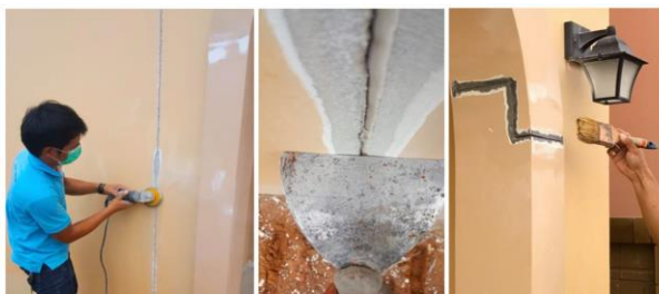
Remove the old jointing material and apply RHINOZ primer bonding.
