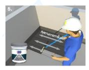
Apply the first coat of 3D Elastic C200 in the same direction by brush or roller, allow it to dry for 2-4 hours (at room temperature).
