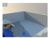
Surfaces must be dry, structurally sound, clean, and free of dust, oil, grease and other contaminants. For cracks and hollow joints must be filled with RF-106 RHINOZ Cement Rapid Filler.
