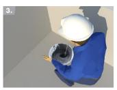
Mix 3D Elastic C200 with the ratio of Part-A:B = 3:1 by weight by low speed mixer (300-500 rpm). Pour 3/4 of powder (Part-A) into a suitable container, add a half of polymer (Part-B) gradually in order to obtain a plastic consistency. Mix in the rest of polymer (Part-B), then add powder (Part-A) and mix until homogeneous before use.
