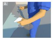
Absorbent substrates must be saturated thoroughly by spraying some water on the desired area and boundary wall up to 10-20 cm above ground level.
