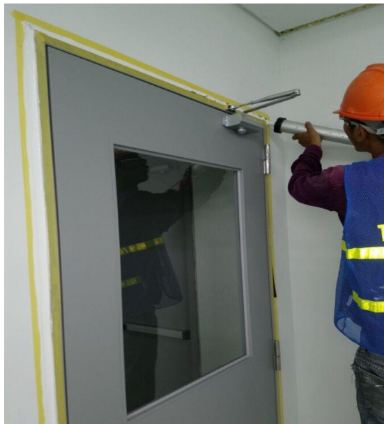
| Trám keo đàn hồi . Sealant application
